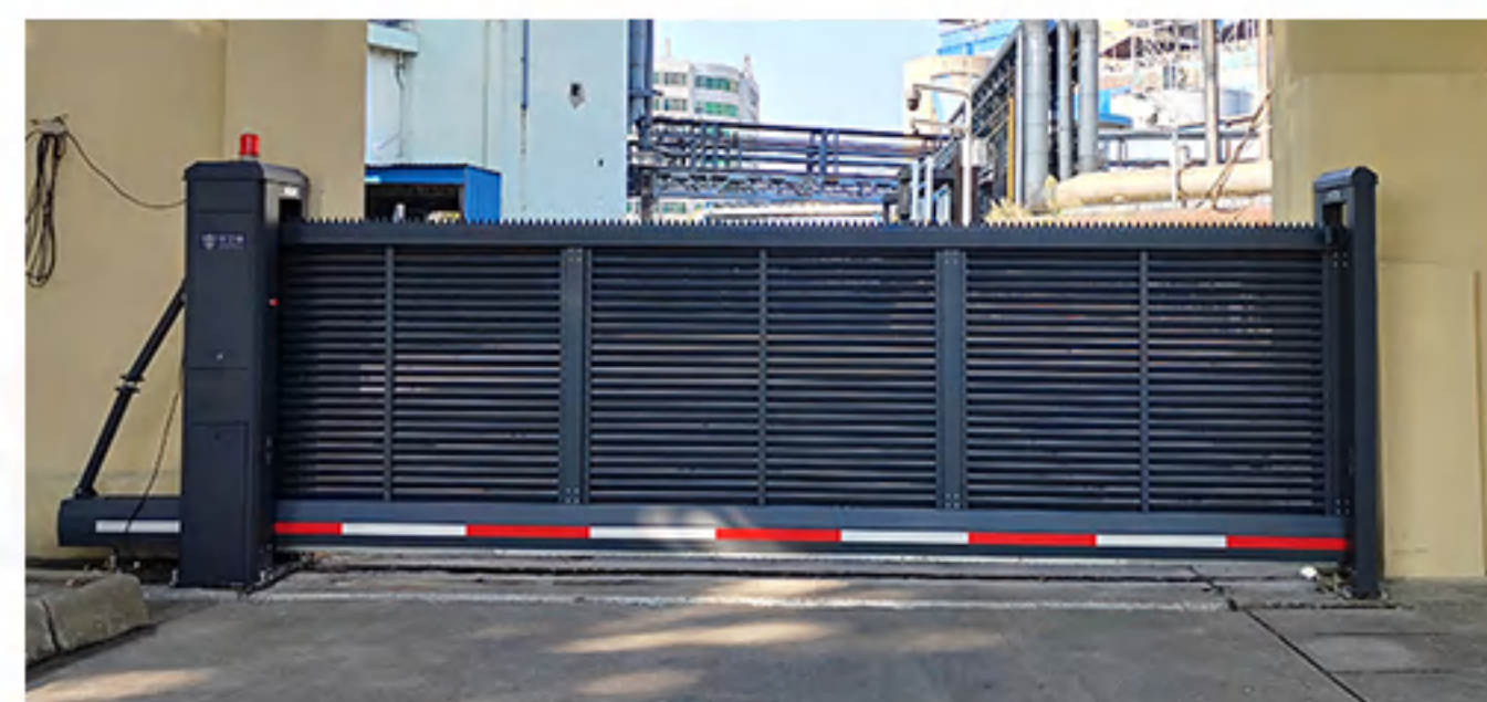
Shanghai Electric Power Service Center
